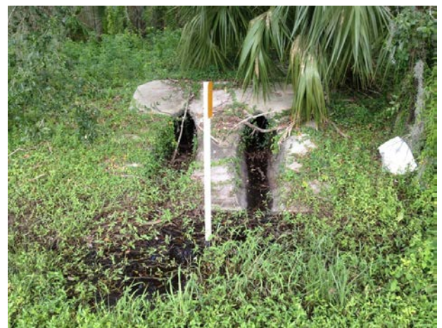
The offsite stormwater pond from the Quail Run RV Resort outfalls into the existing and proposed roadside ditches along I-75.
