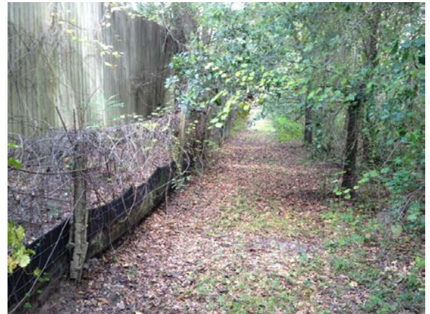
An existing berm prevents offsite drainage flows from the Quail Run RV Resort from entering the FDOT limited-access right-of-way.
